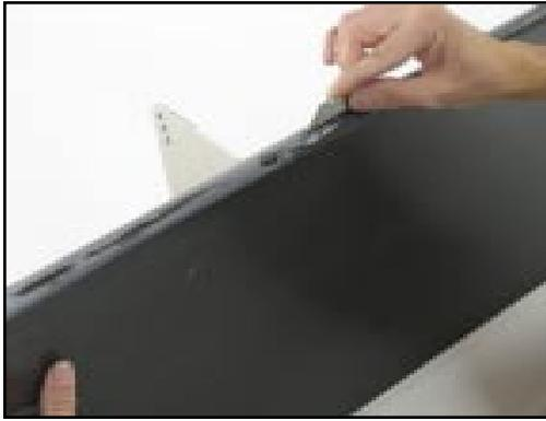
Figure 5. Filling in small pinholes, prior to sanding.
