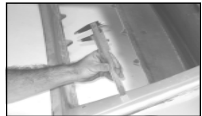
PHOTO 4 Checking Bolt length
